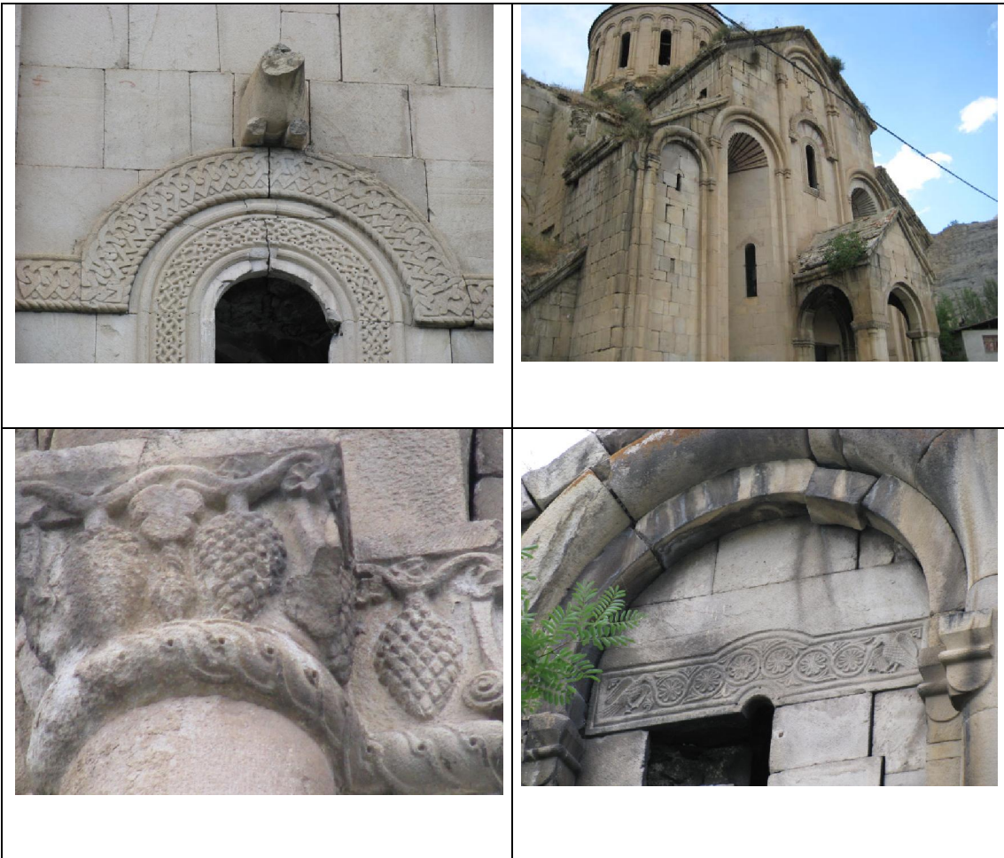
Oshki reliefs, as lace on south facade
